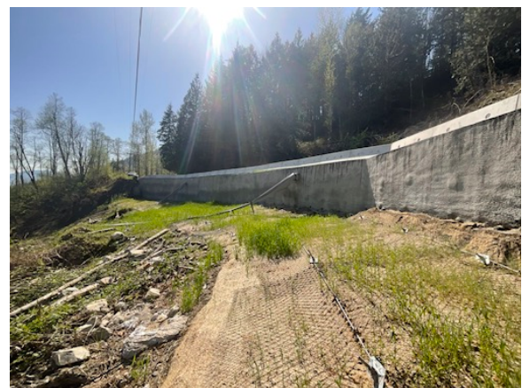
Town side of the wall from woods side
