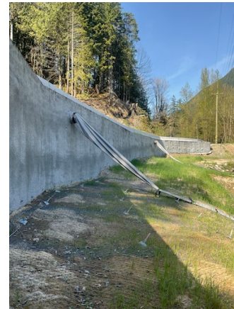
Wall and culvert outlet diversions
